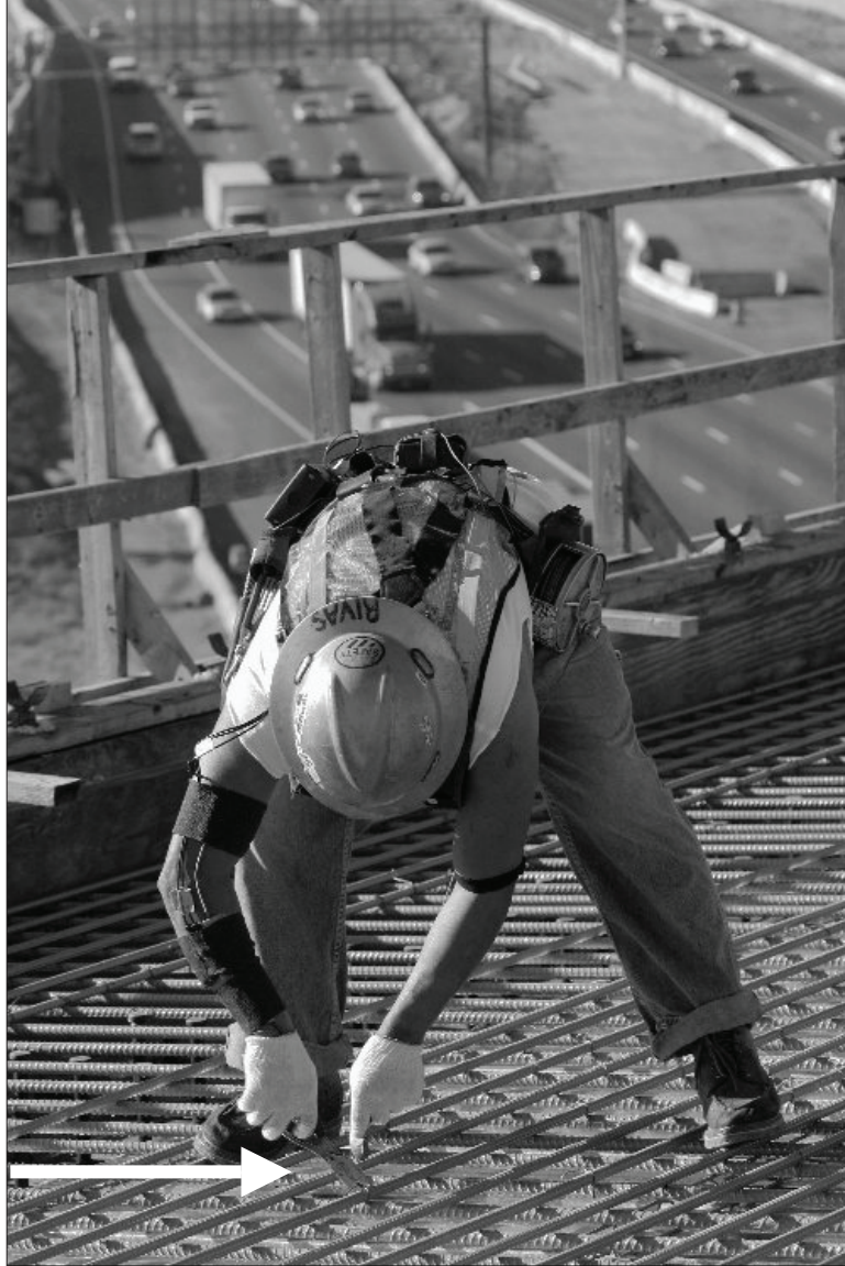
Figure 3 Rebar tying using pliers and tie-wire
